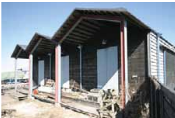
The south end of the lumber storeroom is treated with tar. The other elevations are blue-grey. PM
