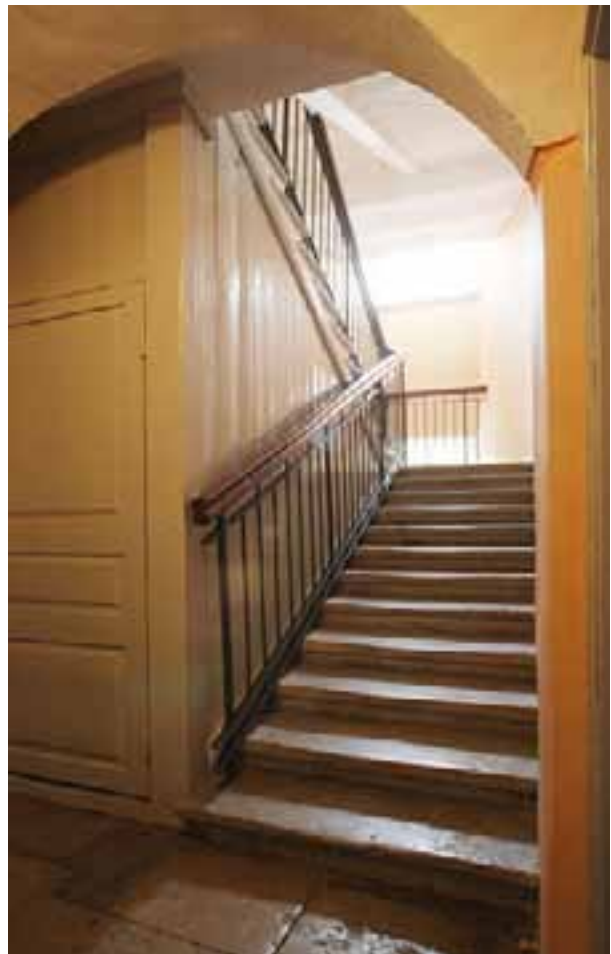
Limestone steps from the late 19th century, staircase C. AdIC
