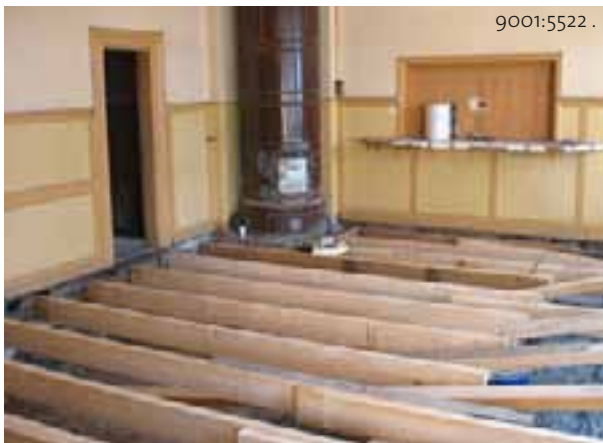
New solid wood beams being installed in the floor of the billiard room. The load-bearing structures of the floors were replaced nearly throughout the building. TK
