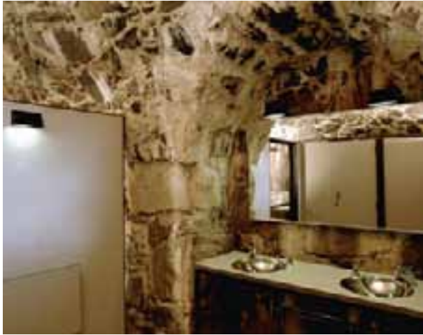
Public conveniences were built in the greystone casemates in bastion Seth so that the new structures stand free of the stone vaults. KJ
