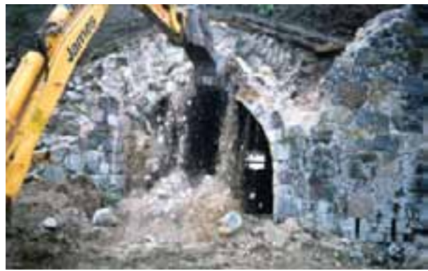
A masonry wall in imminent danger of collapsing was dismantled around an arch which was propped up in hopes that the leaning structure could be preserved and pushed back to its original location using a digger's scoop. This unfortunately proved futile, and the arch was eventually brought down in a controlled collapse.
