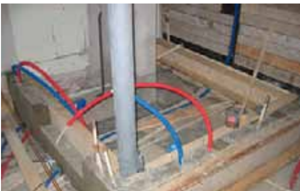
Bathroom installations in the floor structures. KH
