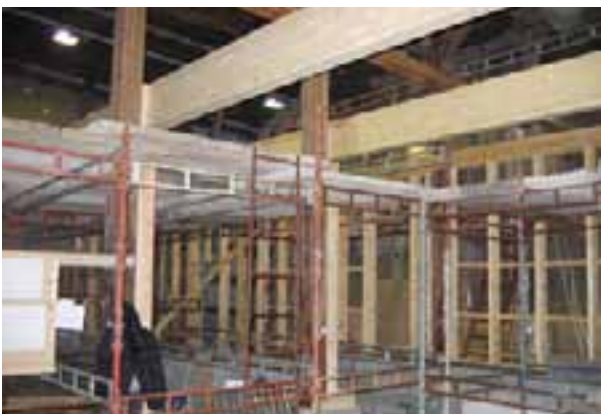
New load-bearing wood pillars were affixed to the existing wood pillars to support the new floor beams, and concrete blocks were used for the interior walls in the wet rooms. RAM
