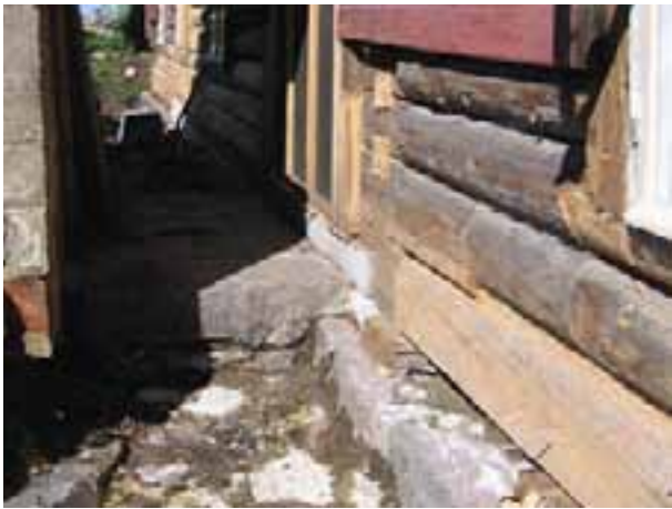
The soil that had accumulated between the building and the adjacent rock face had rotted the lowest logs. The concrete foundation of the cistern is on the left and the original entrance with its stone step on the right. RAM
