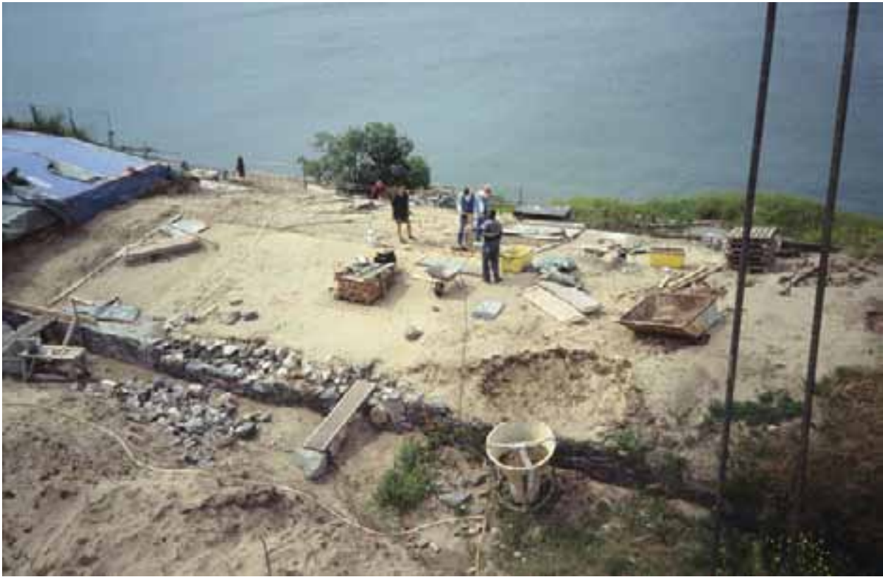
A view from the tower crane to the sand covering of the right flank of bastion Polhem, which is in the process of being waterproofed.
