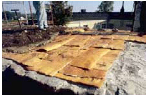
The birch bark and clay waterproofing for the top of the parapet on bastion Gyllenberg was laid in summer 2006. OH
