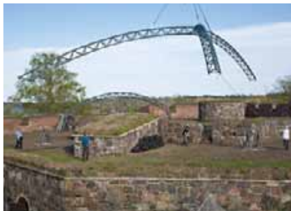
Installation of the load-bearing structures for the new roof in May 2007. JL
