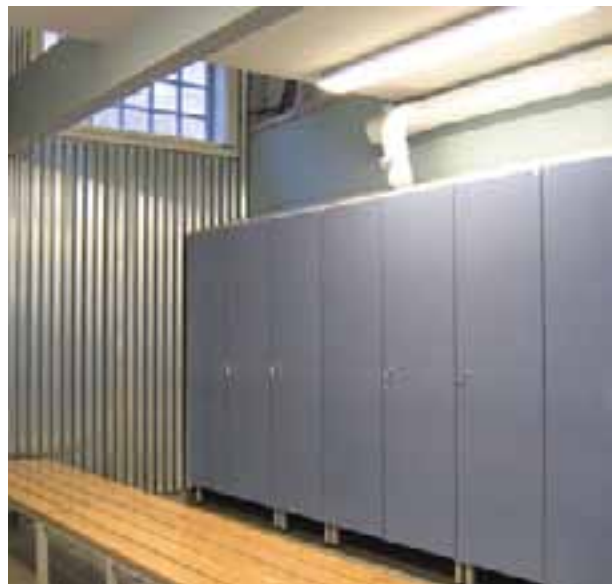
A light shaft was left in front of the windows at the height of the intermediate floor to allow natural light into the changing room. RAM
