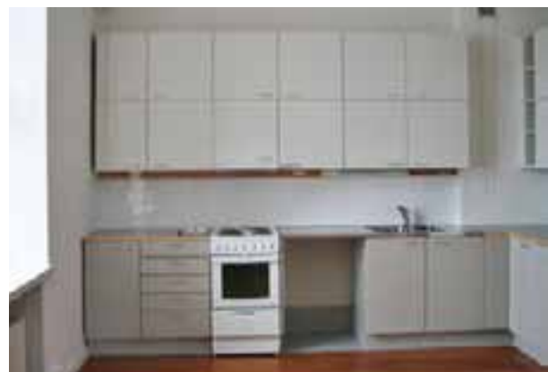
The new kitchen fittings were made of blockboard. LH
