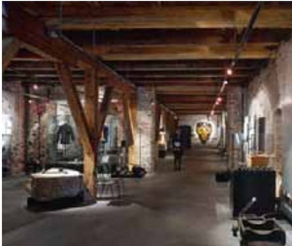
The thick pillars and beams supporting the floor in the old part – partly replaced and partly repaired (lower photo) – and the floor boards (upper photo) were left exposed. VN
