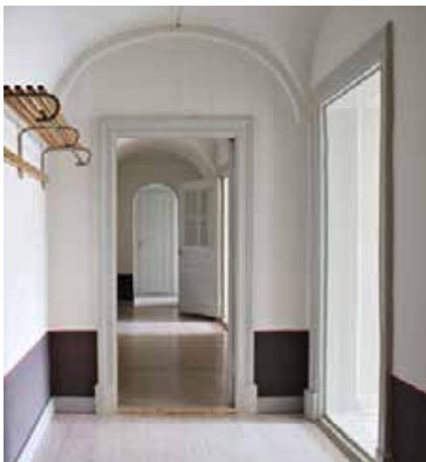
The wall in the front hall is decorated with a dark, splash-pattern 'lamp-black dado' in tempera, outlined in red. The old floor was given a translucent grey glaze. AdIC
