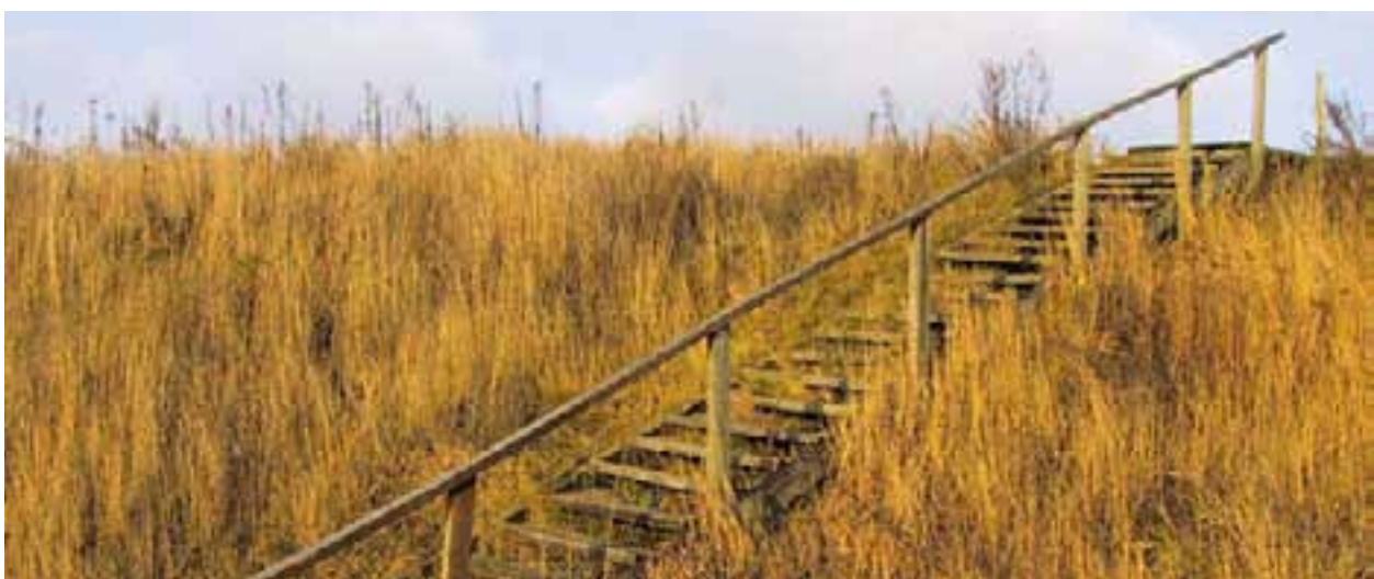
Repairing the earthworks on Suomenlinna and making them more resistant to wear and tear take up an increasing amount of the Governing Body's time. The photo shows a decayed staircase in Battery 4 on Kustaanmiekka; this was replaced in 2000. PN
