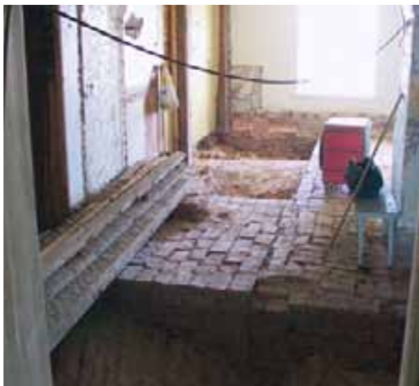
The ceilings of the lower floors are brick-vaulted, those of the upper floors wooden. RAM
