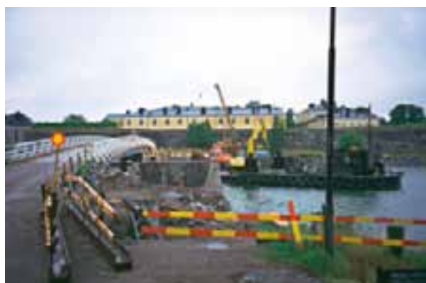
The new Pikku Mustasaari bridge was first built alongside the old bridge, which was then dismantled. New piers were built on the location of the old bridge, and the new bridge was finally moved onto the new piers in the course of a single working day. KH
