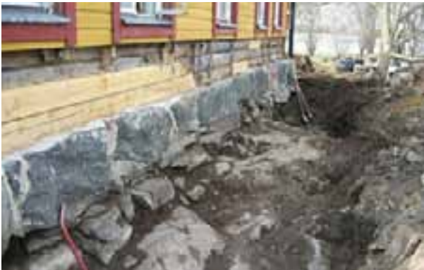
The old foundation wall was repaired by putting displaced stones back in place. The photo also shows some of the repaired log wall on the eastern side. KH
