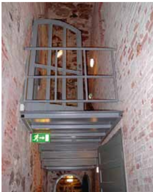
An emergency exit was built on the top floor by enlarging an old ventilator, making an opening in one of the brick walls of the flanking corridor, and building four flights of steps and four landings. KH
