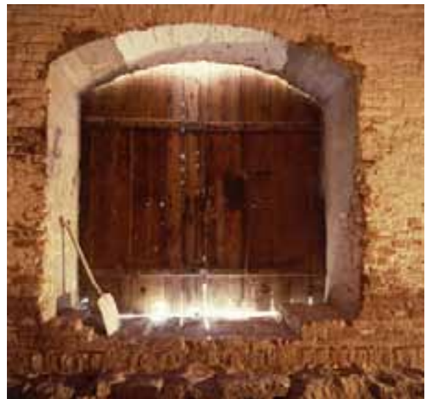
The vaulting in the doorway clearly shows where the doorway has been widened. MK
