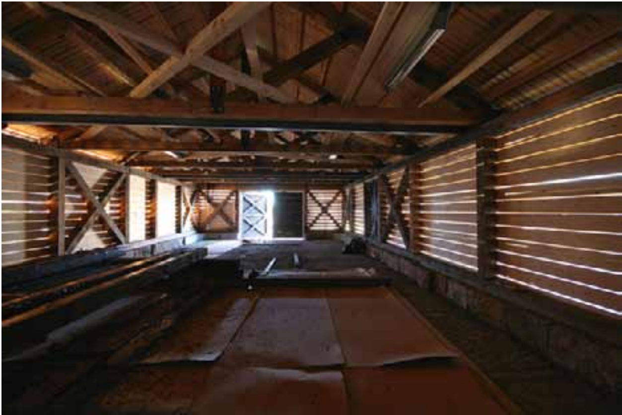
The weatherboarding was designed to allow air to pass through. PM
