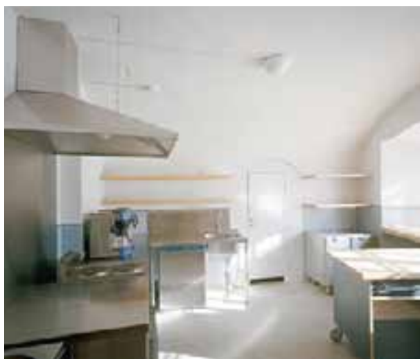
The small kitchen adjacent to the mill hall was built in an intermediate space that had undergone numerous alterations. The mill hall, kitchen and toilets have mechanical extractor fans, though elsewhere the ventilation is natural. JT
