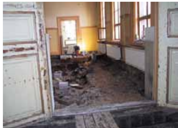
The floor structures being dismantled. TK
