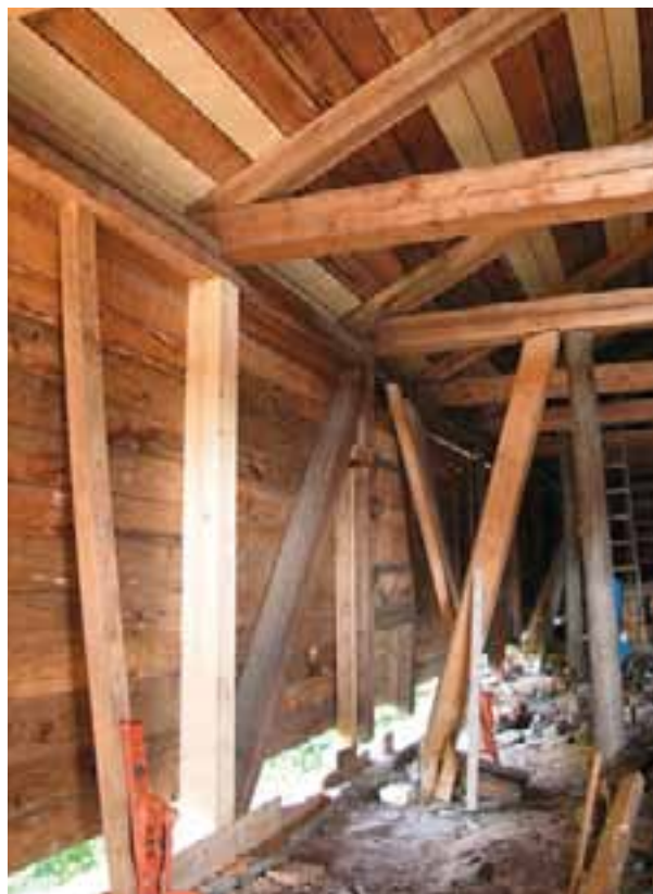
The wall was jacked up so that logs could be replaced. KH
