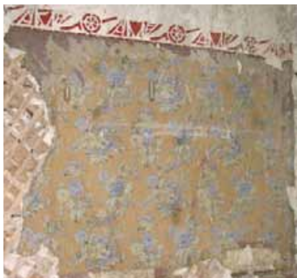
The Governing Body of Suomenlinna conservators carefully examined and documented the numerous layers of paint and wallpaper on the walls. RAM
