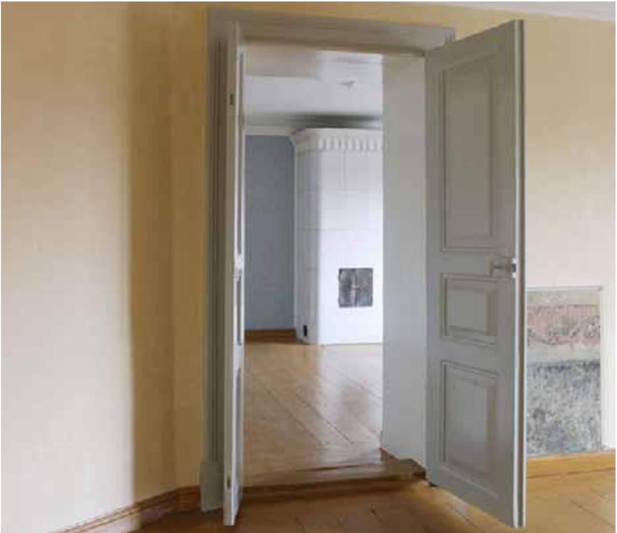
The old wood floors are painted yellow ochre to match the oldest paint layer uncovered in the colour examinations. The wallpaper was chosen to match the late 18th-century colour scheme. AdIC
