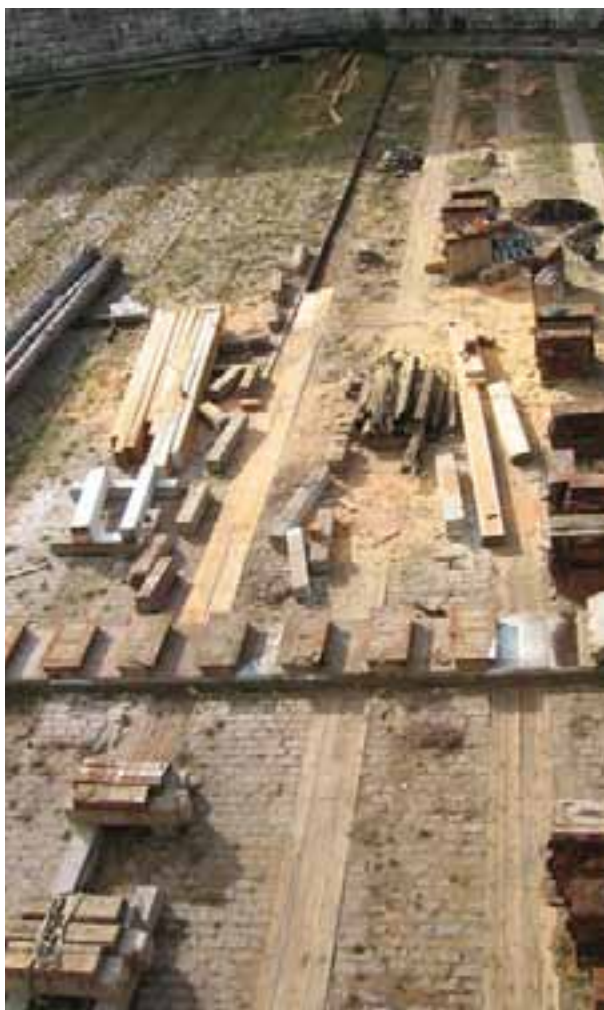
Replacing the bottom timbers in the dock basin. Besides major repairs the dock structures require continuous maintenance.
