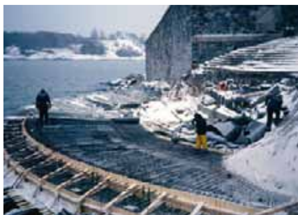
Laying the reinforcing irons for the new quay slab in December 1997. TL
