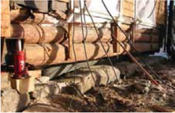
The lowest timbers in the outside walls were replaced. KH
