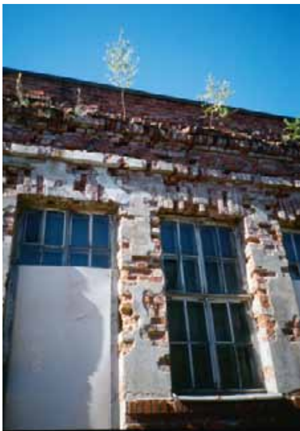
The brick elevations of the former mine workshop (C 34) were in extremely poor condition when repairs began.
