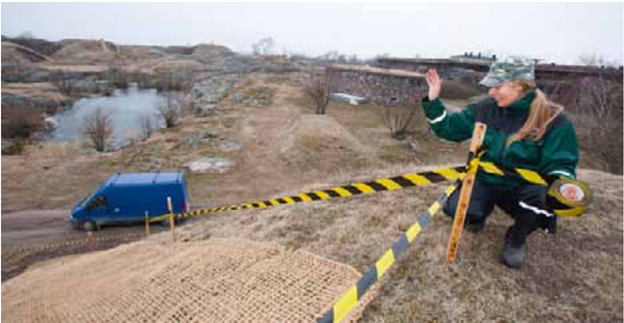
Gardener Iina Johansson repairing erosion damage to the earth covering of a powder magazine on Kustaanmiekka. EJ
