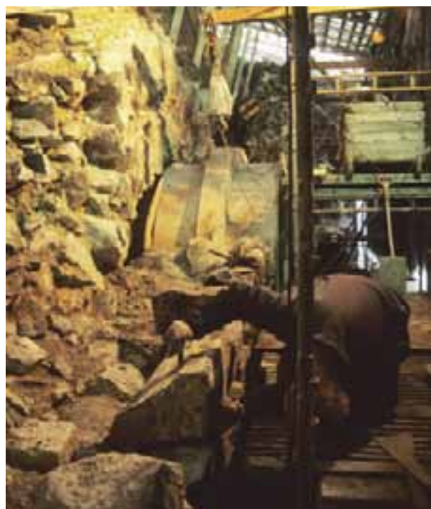
Reconstructing the dismantled arch and surrounding wall in winter conditions. MV
