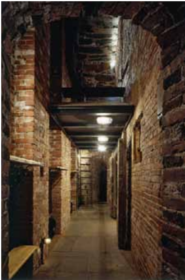
Coat racks and a steel-built balcony for AV equipment were built in the narrow circling corridor at the south end. JT
