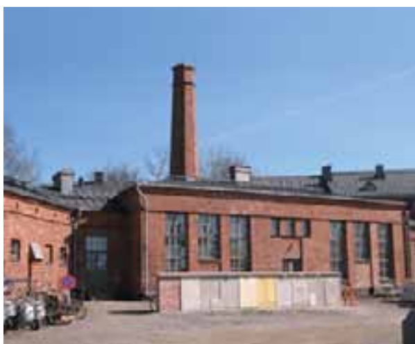
The yard side windows in the construction office were extended downwards, and the garage door, a later addition, was restored to two windows (on the right in the photo). In the foreground is a brick wall erected for weather-testing lime mortars. PM
