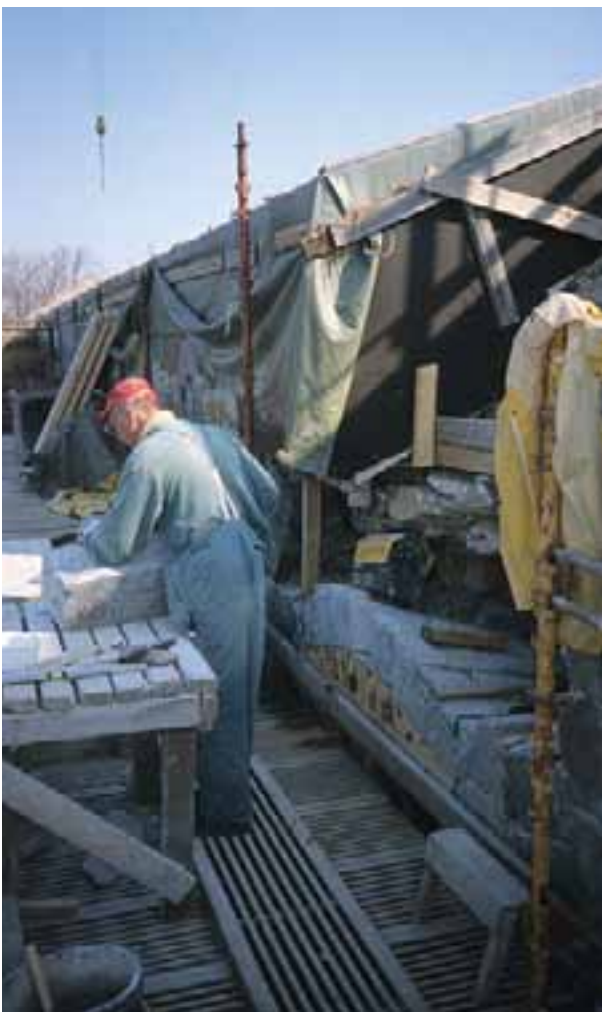
Replacements for vaulting stones missing from a collapsed embrasure being manually dressed in Kuru gray granite. TL
