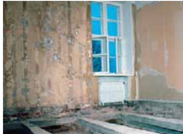
The concrete floor slab structure built in the 1930s exposed during the repairs.
