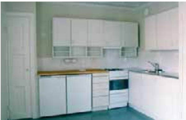
New lower cupboards were installed to complement the old, reconditioned kitchen fittings. Building E 3. SW
