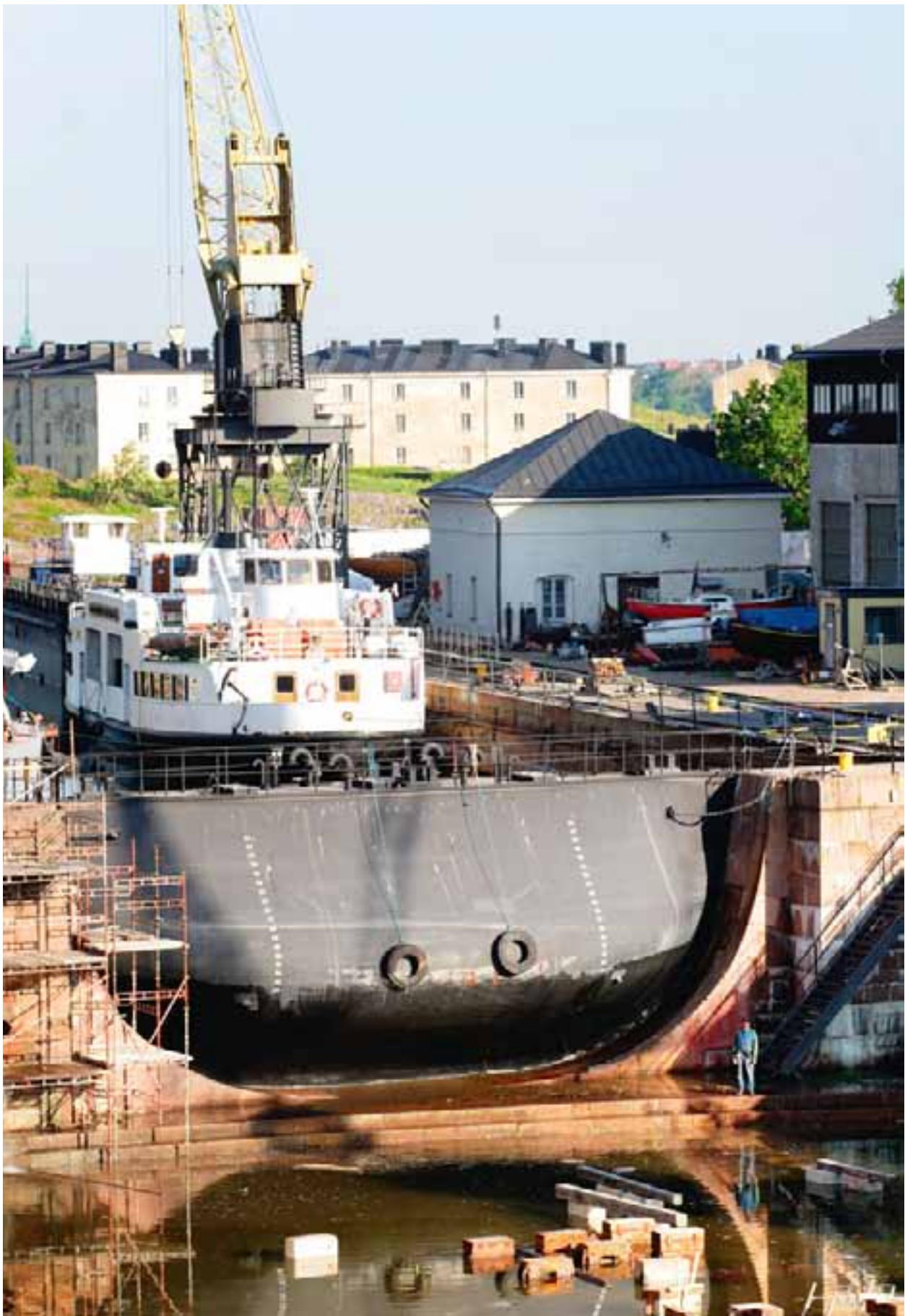
The two dock basins are separated by an intermediate lock gate, thanks to which vessels can be docked in the outer basin without filling the inner basin with water. The original intermediate lock gate dated from 1862; it was replaced in 2004. MRa
