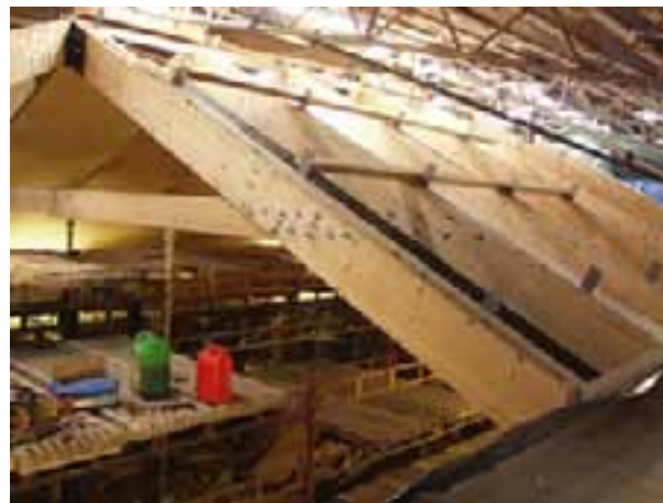
Roof rafters being installed in winter 2005. PM
