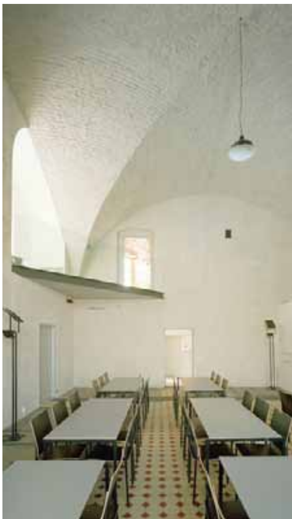
The mill hall, a large cross-vaulted space, was originally divided into two storeys by a wooden intermediate floor. The modern steel-and-glass platform that leads to the rear rooms on the second floor marks the location of the dismantled floor. JT
