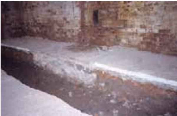
An installation duct for water mains, sewers and heating pipes was cut in the old flooring which was preserved. The base of an old fireplace can be seen in the middle. TL
