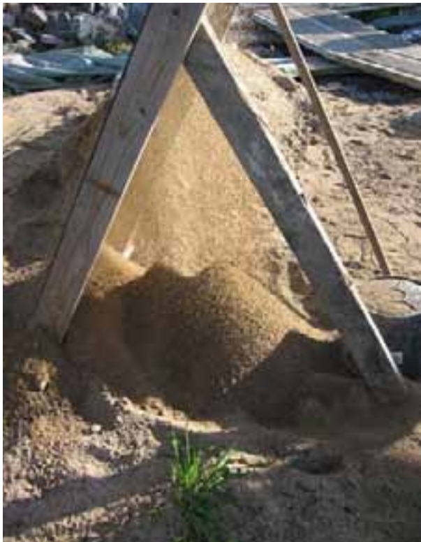
The maximum grain size of the sand used for mortar is 8 mm. For grouting, the sand is sieved manually at the work site using a 6 mm sieve. KH
