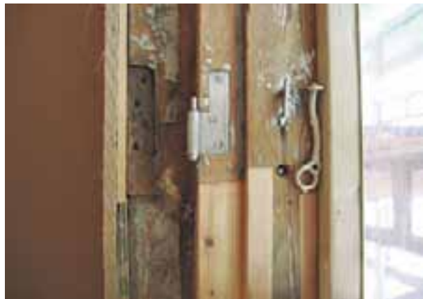
The window frame spline shows a trace of the original window or the hinge of a window shutter. The current windows were probably made in the 1930s. RAM
