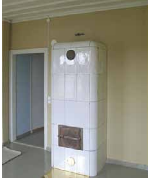
A re-erected tiled stove in the sitting room. TK
