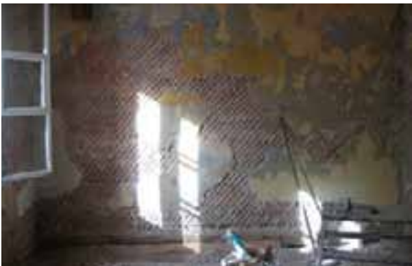
The plasterwork in the kitchen before repairs. TK
