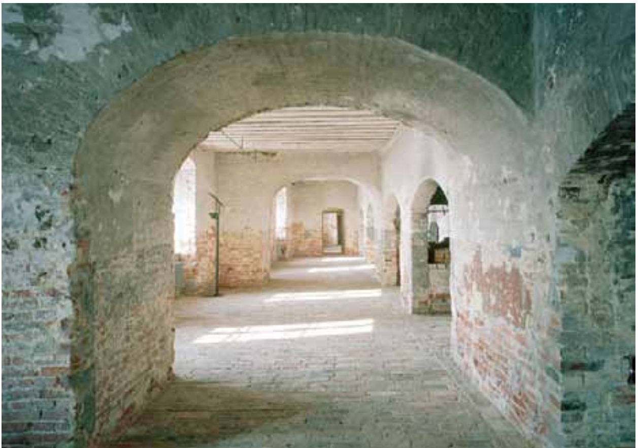
The bakery contains six large baking ovens built for provisioning the Archipelago Fleet. The new floor was made of bricks from a dismantled structure elsewhere and built to the level of the original brick flooring, which had been dismantled in the 1960s. The paintwork on the walls was conserved. JT
