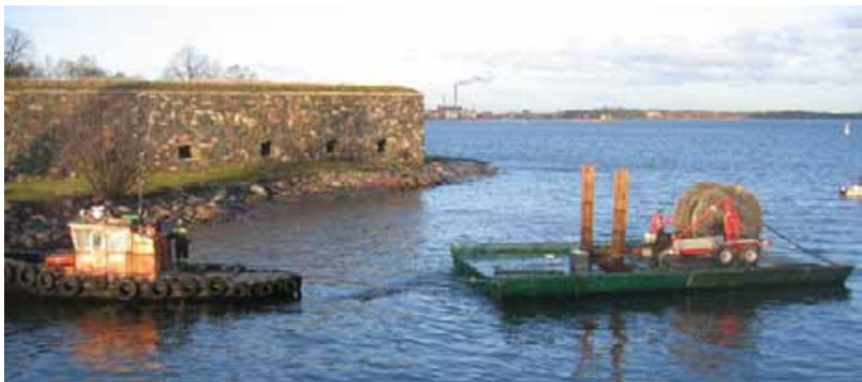
Electrical cable being laid between Lonna and Pikku Mustasaari islands in December 2007.
