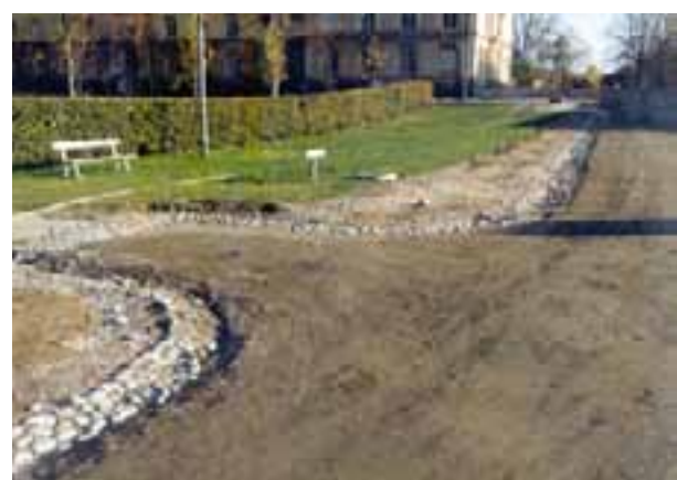
Laying macadam paving in autumn 1996. The aggregate layers are watered and then rolled to compress them into a solid surface. Moraine is spread on top as a binding agent. PN
